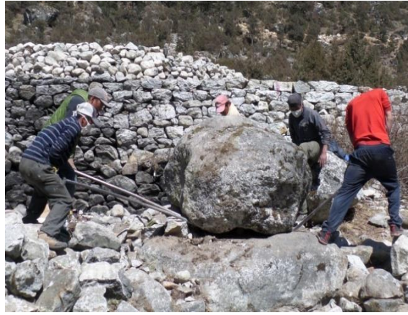
PREPARING STONE FENCE
