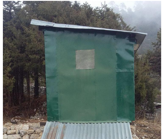
NEWLY IMPROVED REST HOUSE (TOILET)
