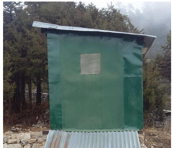
NEWLY IMPROVED REST HOUSE (TOILET)
