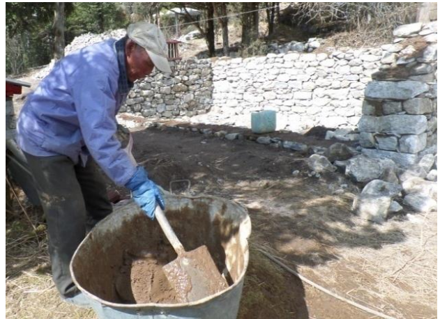
USING YAK DUNG TO PLASTER THE WALLS
