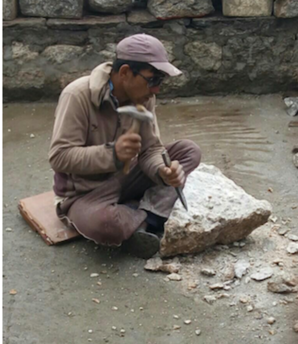
Figure 11: Worker shaping stone into appropriate shapes required for construction
