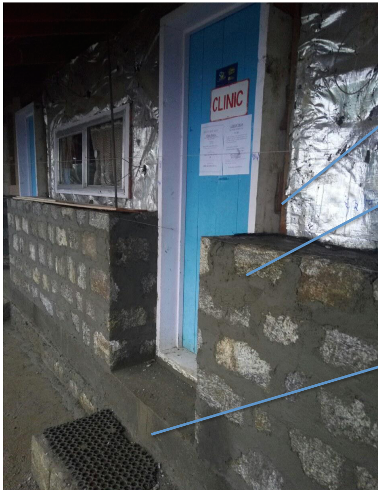
Figure 12: Building stone masonry wall with cement mortar as suggested in the design. It is currently ongoing and reached just below the sill tie level.
