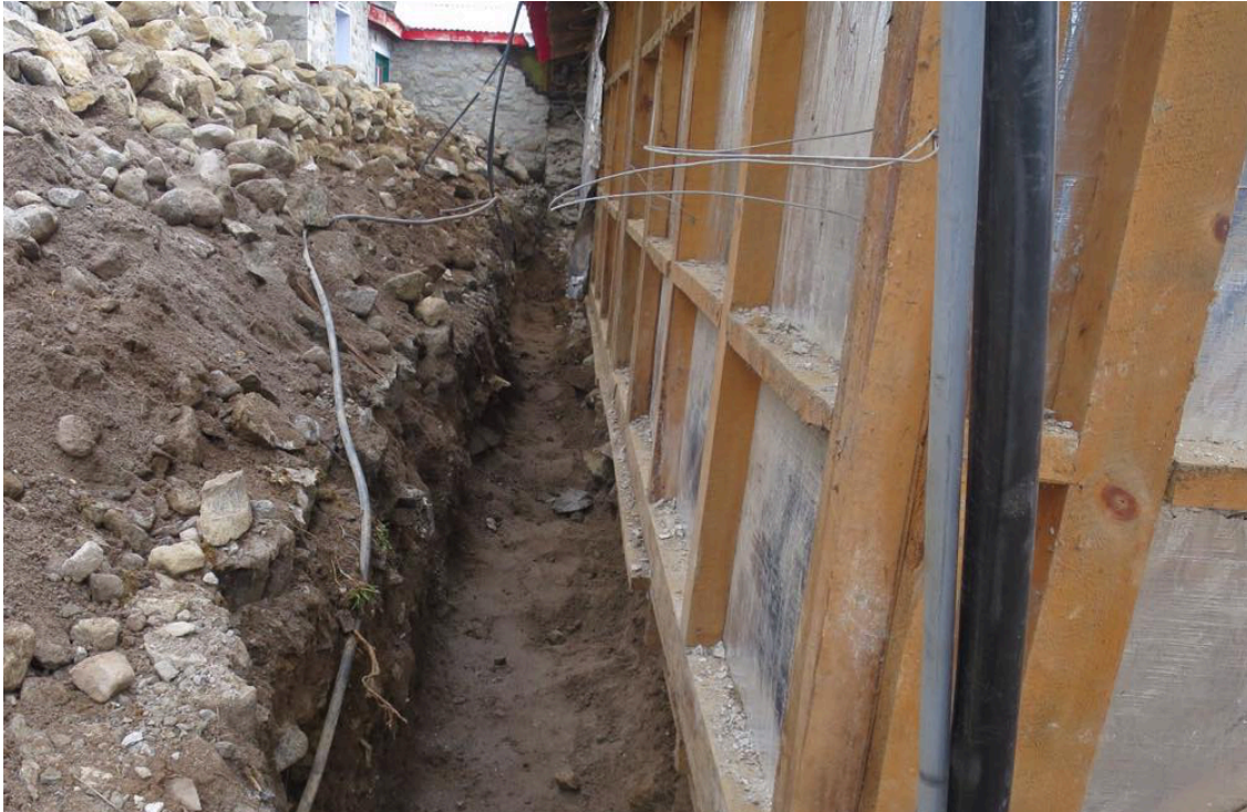
Figure 5: Surprisingly, there was no foundation in the older structure. The rock wall of the building has been constructed above ground level. Thus, a new 3 feet depth and 2.5 feet width foundation was dug as per the instructions provided in the engineering design
