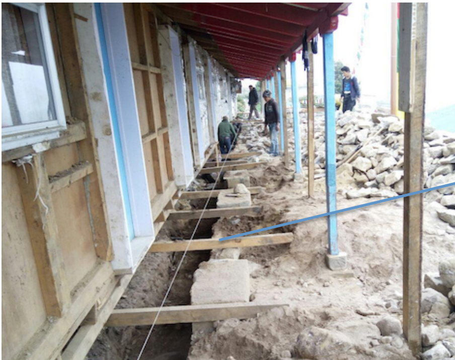
Figure 4: Wooden support system was setup for supporting the internal structure at the bottom, side, back and front (in picture) of the building during the construction.
