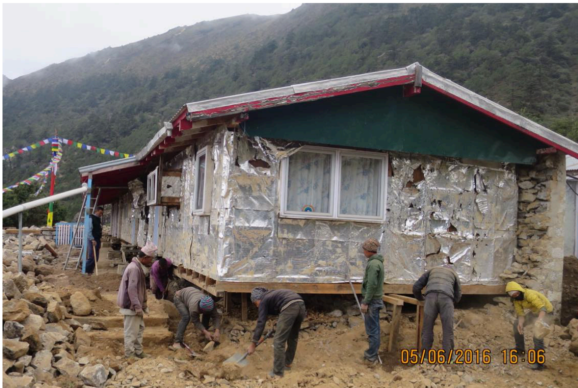
Figure 1: The main hospital block after demolishing the external rock wall
