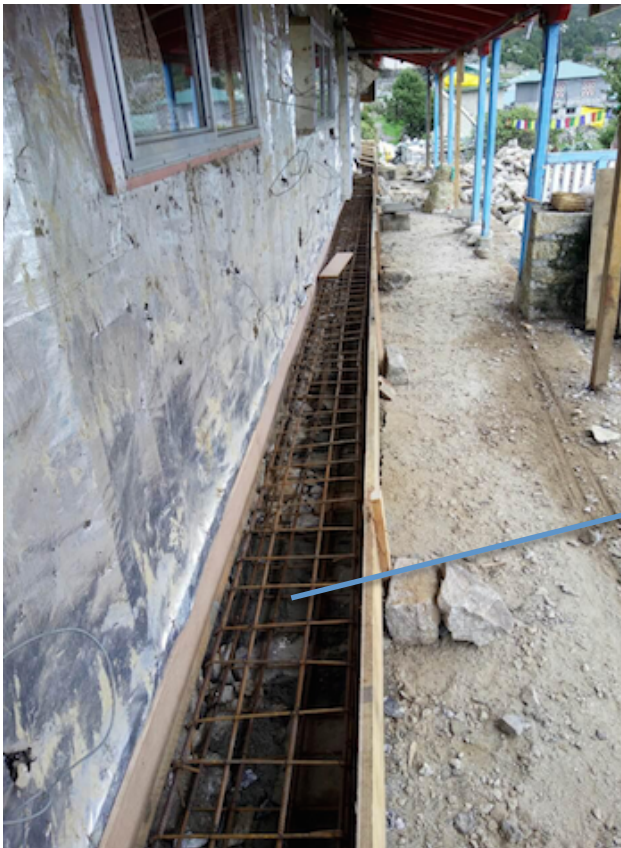
Figure 8: D.P.C. tie beam placed horizontally all round the building above the ground level. The D.P.C is 9-inches in height and 18-inches in breadth.
