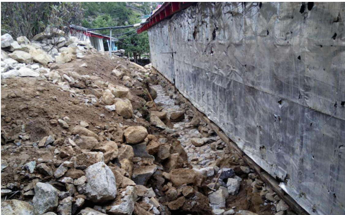
Figure 6: Stones and cement has been used in the new foundation. Cement was not mentioned in the engineering design, but has been used to make it firmer as suggested by the engineers recently. Since there was no foundation in the previous structure, most of the stones were used in foundation. Luckily, we got 6 strong stonebreakers to break more stones, thus everything has been running smoothly.
