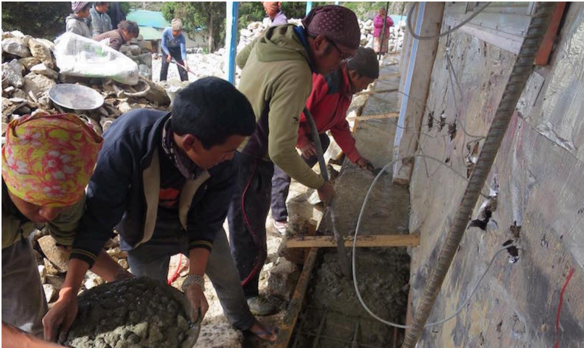
Figure 10: Spreading and compacting cement mortar in the D.P.C. layer with a machine.
