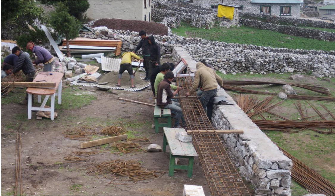
Figure 7: Workers weaving a D.P.C. tie beam with varied diameter iron rods following the instructions provided in the engineering design.
