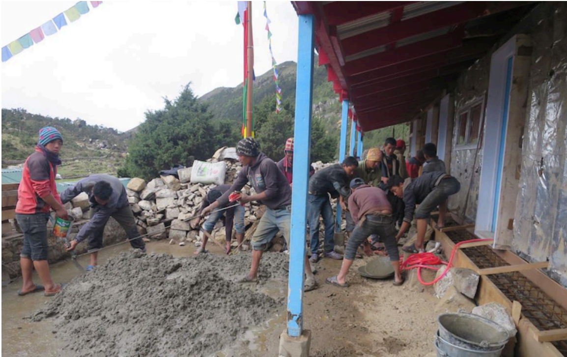
Figure 9: Workers making cement mortar combining a mixture of sand and cement for D.P.C.
