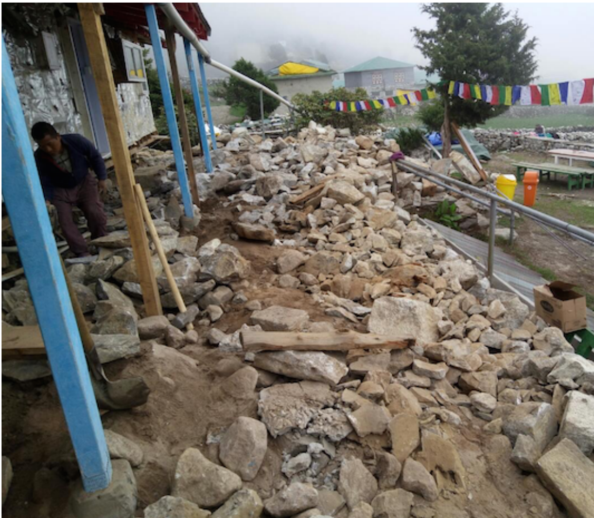
Figure 2: The outer rock wall structure of the building was scraped and demolished keeping the internal wooden structure intact.
