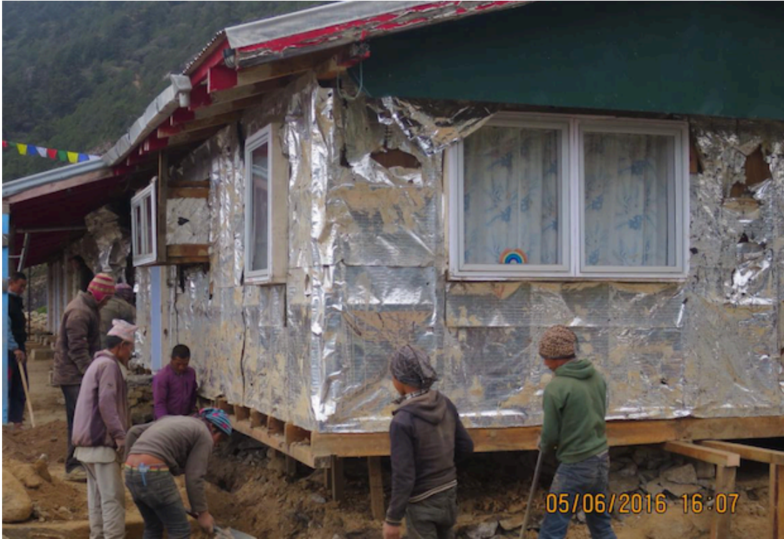
Figure 3: The main hospital block after demolishing the external rock wall. Demolishing and site clearance work has been completed within few days. The outer silver cover is the insulation material, which has been kept intact.
